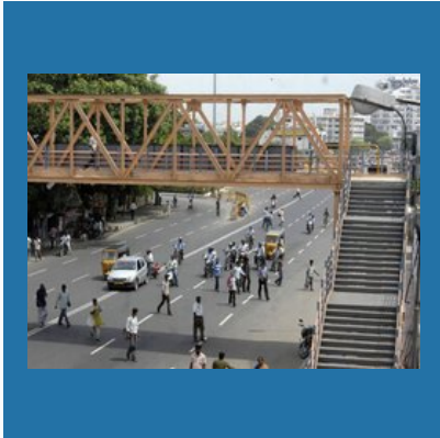
Foot Overbridge Construction Services
